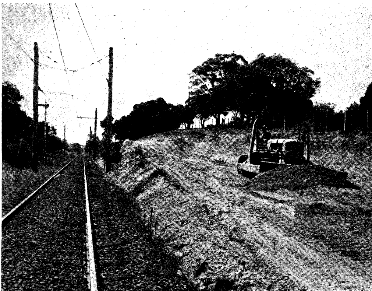
Duplication Work on the Ashburton Line.
